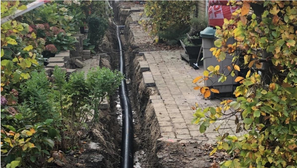
Figure 3. Installation of the service pipes in Østerby district
